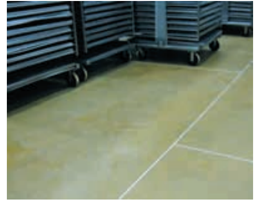
The Sika floor installation was completed within a very tight timeframe
