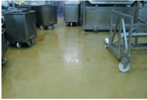
Floors were finished with a durable slip-resistant finish to ensure maximum safety for staff
