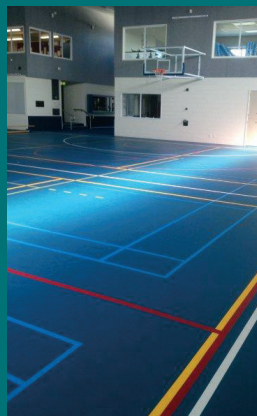
A self-smoothing layer of seamless Pulastic floor is then applied.
