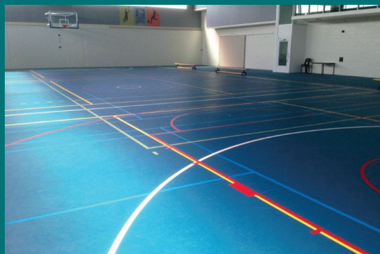
A final Pulastic top coat is applied and then the customised markings are added.
