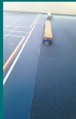
A self-smoothing layer of seamless Pulastic floor is then applied.
