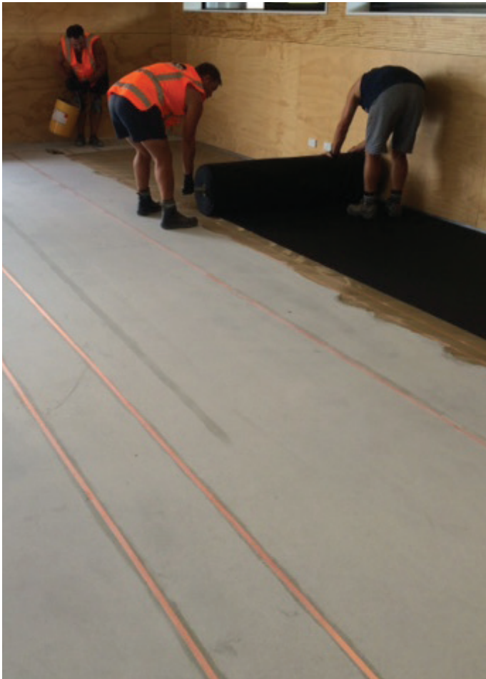
Placing the shock absorbing mat
